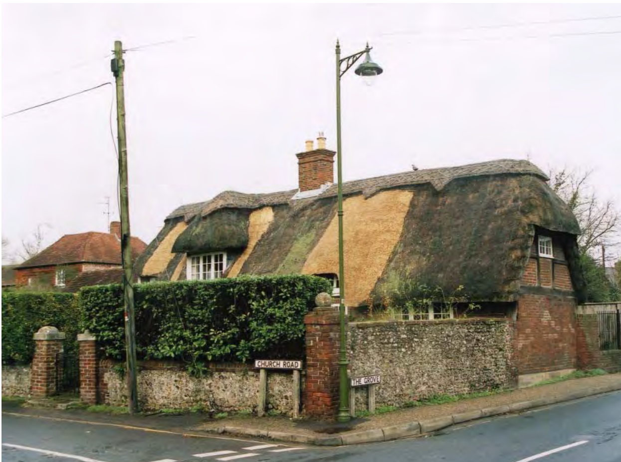
Overhead cables in Church Road
