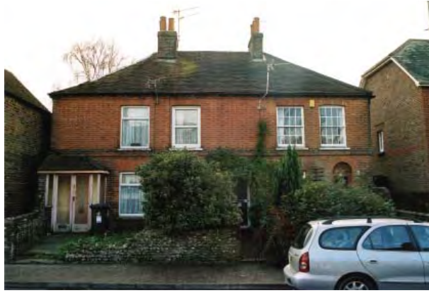
Non designated heritage assets can easily be harmed by the incorrect use of modern materials such as UPVC window frames
