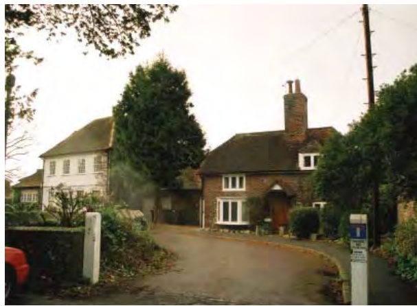
Entrance to Old Rectory Close
